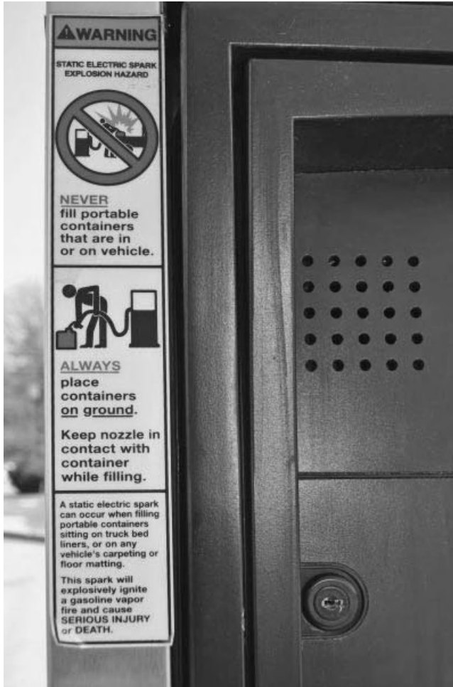
Figure 4.11 Gas pump ESD warnings
